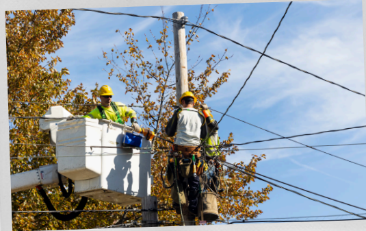
Leading the nation in clean energy
